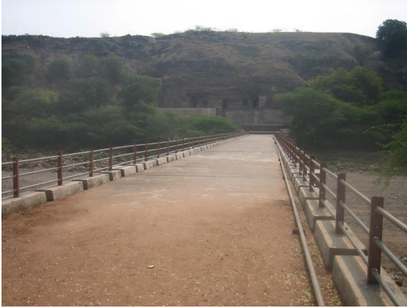
114 Bridge to Bagh Caves, Madhya Pradesh, late fifth century
