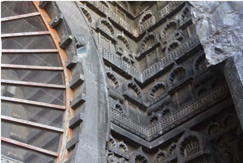
48- End wall of verandah, chaitya hall, Karla Caves, Maharashtra, 120 AD
